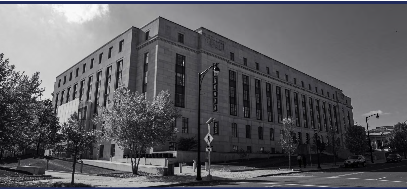
APA Central Office State Office Building - 165 Capitol Avenue, Hartford, Connecticut
